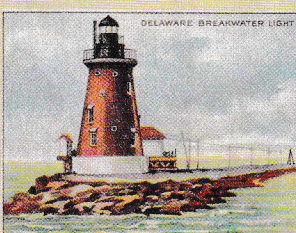
DELAWARE BREAKWATER LIGHT
