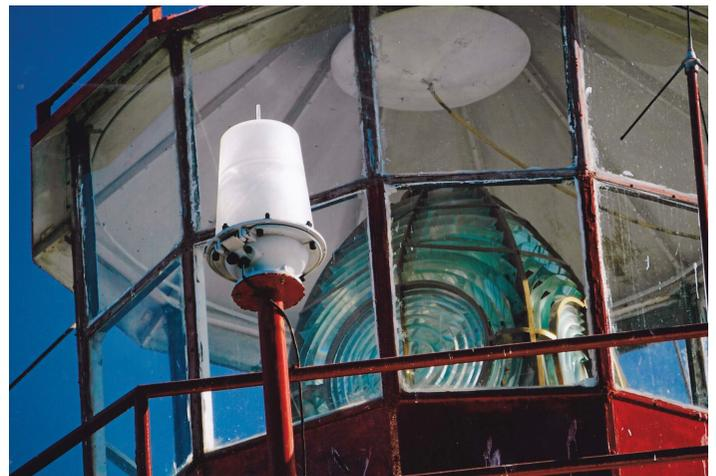
The old Fresnel lens in the lantern at El Faro is still in use.
